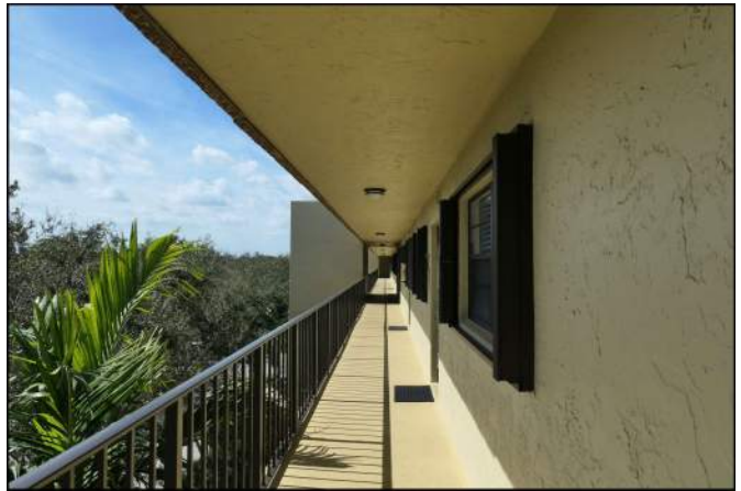
Photo 58 Building Structure and Envelope
