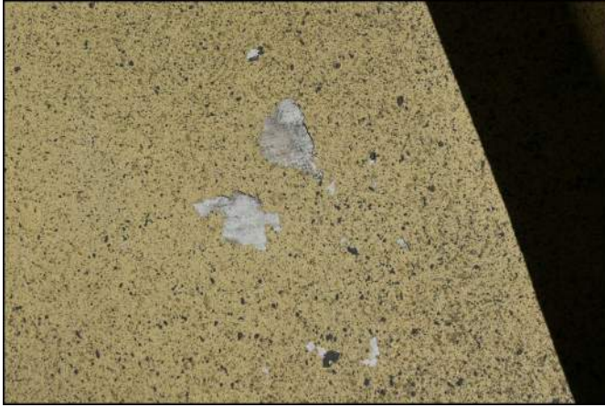
Photo 37 Building Structure and Envelope
