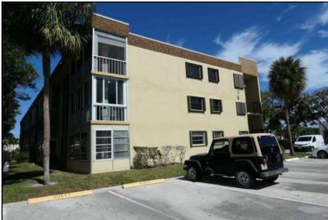
Photo 33 Building Structure and Envelope
