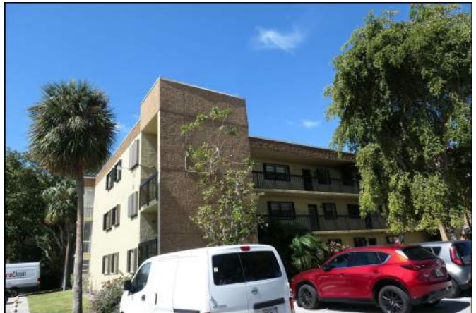
Photo 34 Building Structure and Envelope
