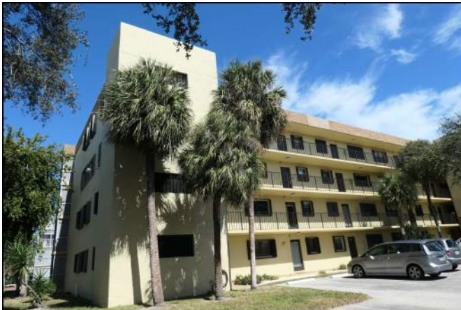
Photo 51 Building Structure and Envelope
