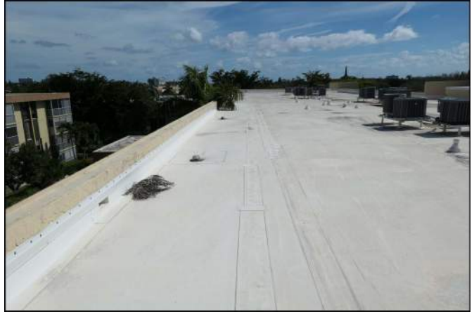
Photo 50 Building Structure and Envelope
