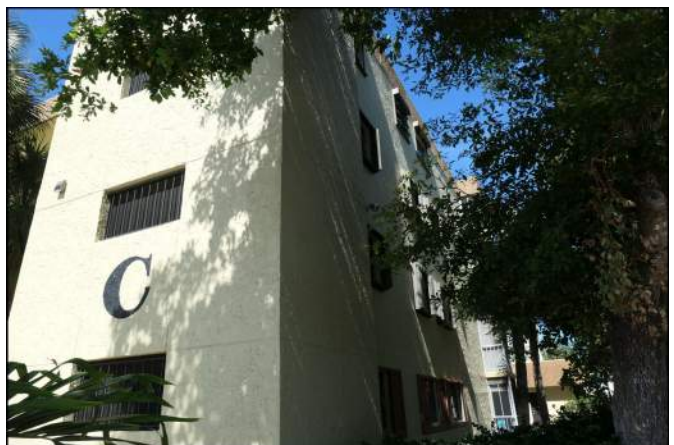
Photo 54 Building Structure and Envelope
