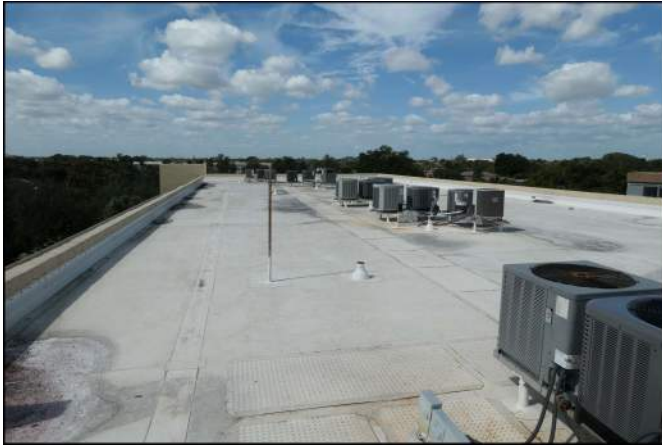
Photo 45 Building Structure and Envelope
