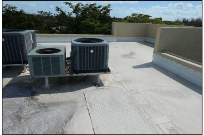
Photo 46 Building Structure and Envelope
