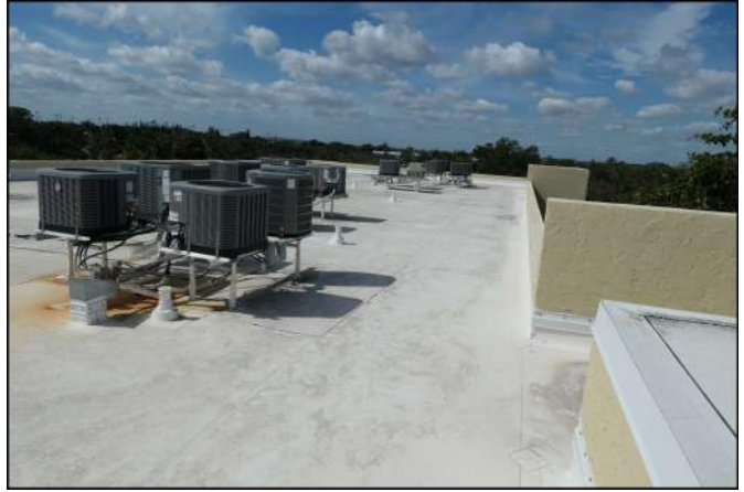
Photo 02 Building Structure and Envelope
