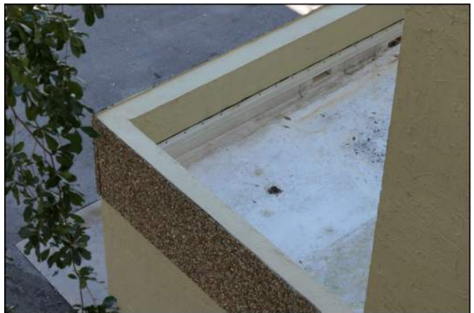
Photo 24 Building Structure and Envelope
