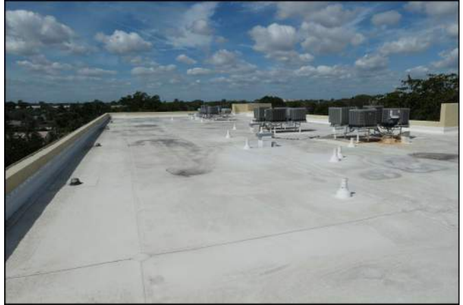
Photo 08 Building Structure and Envelope
