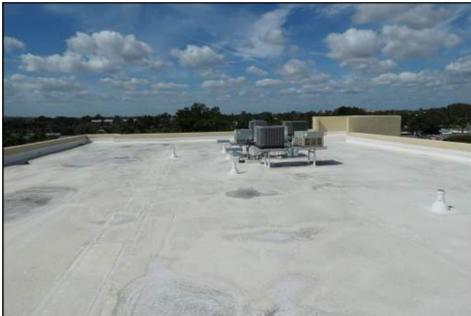
Photo 09 Building Structure and Envelope
