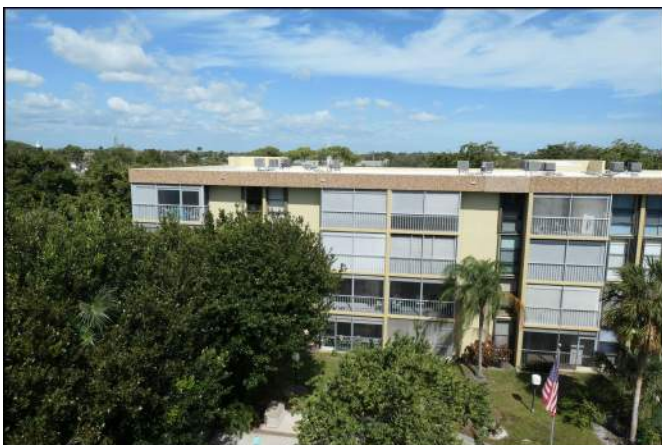
Photo 11 Building Structure and Envelope
