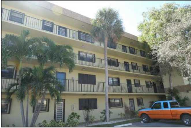
Photo 13 Building Structure and Envelope
