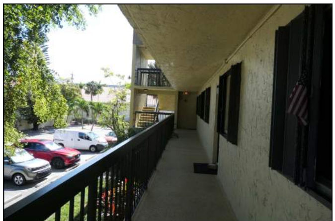
Photo 36 Building Structure and Envelope
