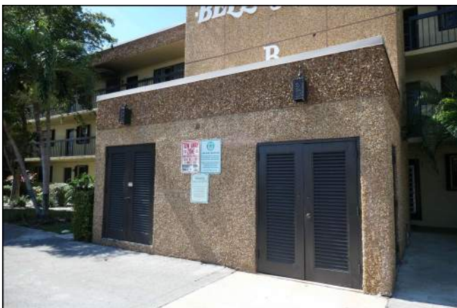
Photo 35 Building Structure and Envelope
