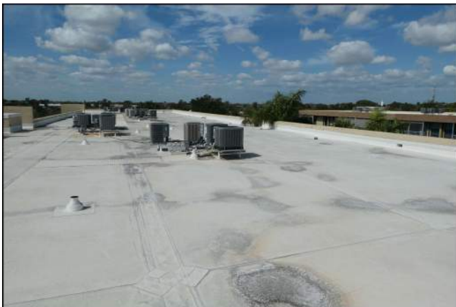
Photo 47 Building Structure and Envelope
