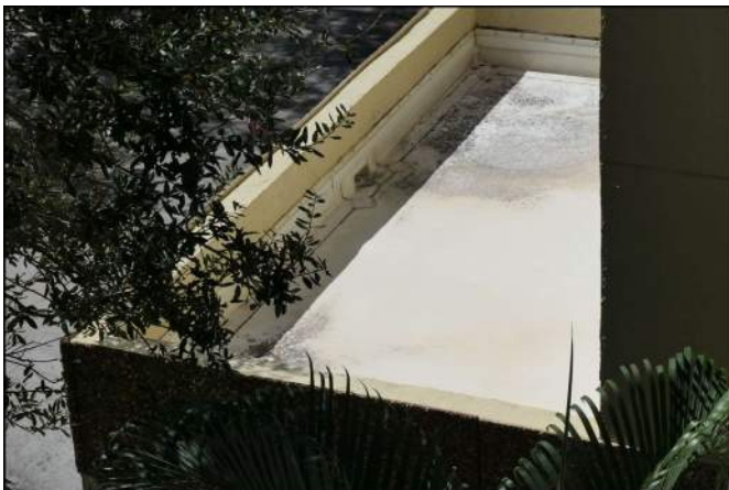
Photo 59 Building Structure and Envelope
