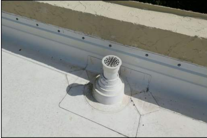
Photo 07 Building Structure and Envelope
