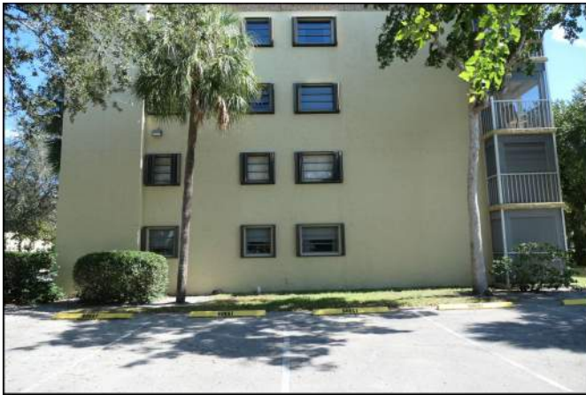
Photo 15 Building Structure and Envelope
