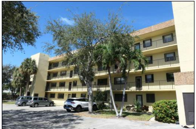
Photo 52 Building Structure and Envelope
