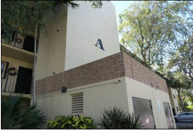
Photo 01 Building Structure and Envelope
