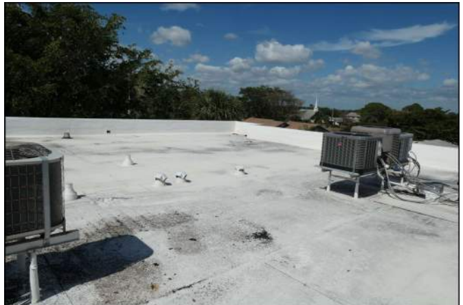
Photo 28 Building Structure and Envelope
