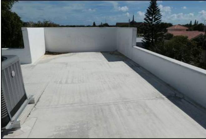
Photo 31 Building Structure and Envelope
