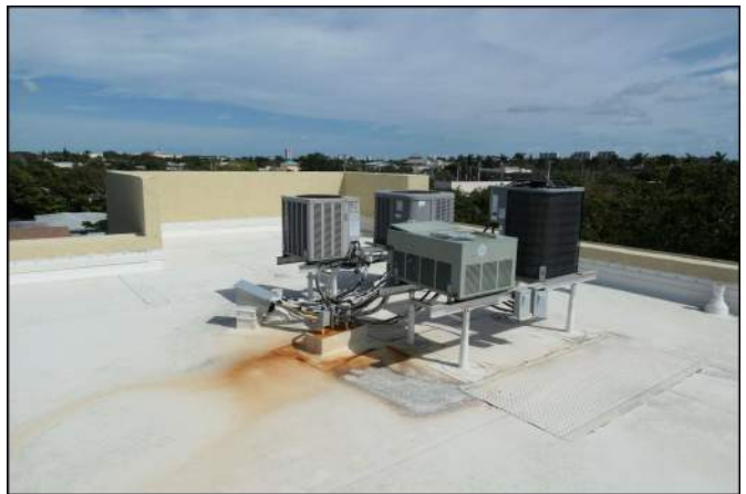
Photo 06 Building Structure and Envelope
