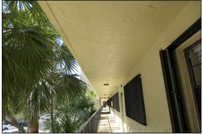
Photo 56 Building Structure and Envelope
