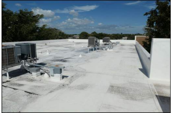
Photo 26 Building Structure and Envelope
