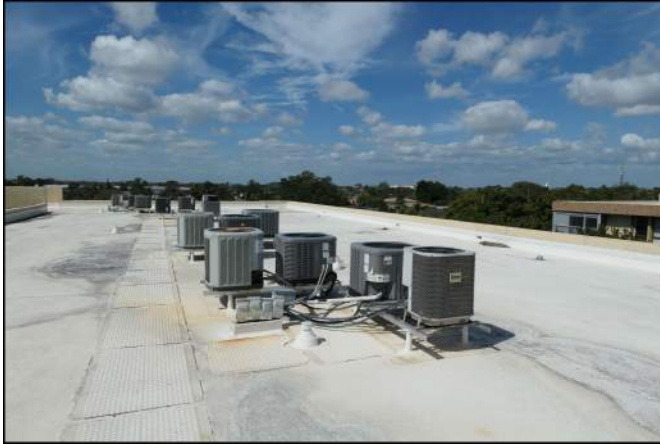
Photo 49 Building Structure and Envelope
