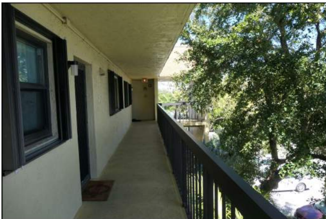
Photo 41 Building Structure and Envelope
