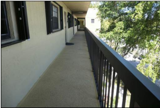
Photo 39 Building Structure and Envelope
