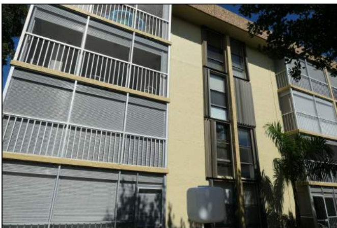
Photo 17 Building Structure and Envelope
