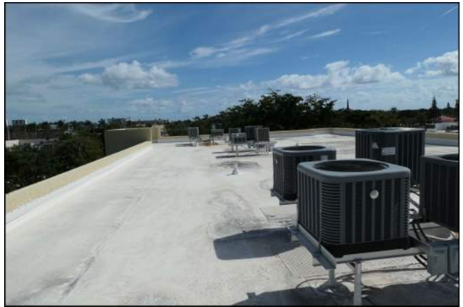
Photo 04 Building Structure and Envelope
