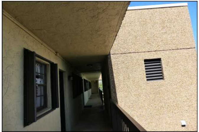
Photo 40 Building Structure and Envelope
