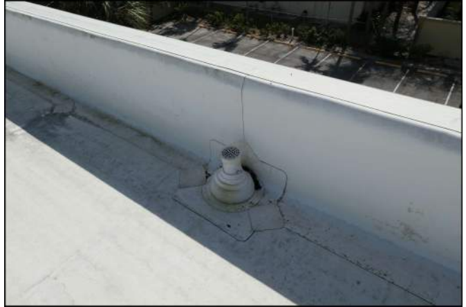
Photo 32 Building Structure and Envelope
