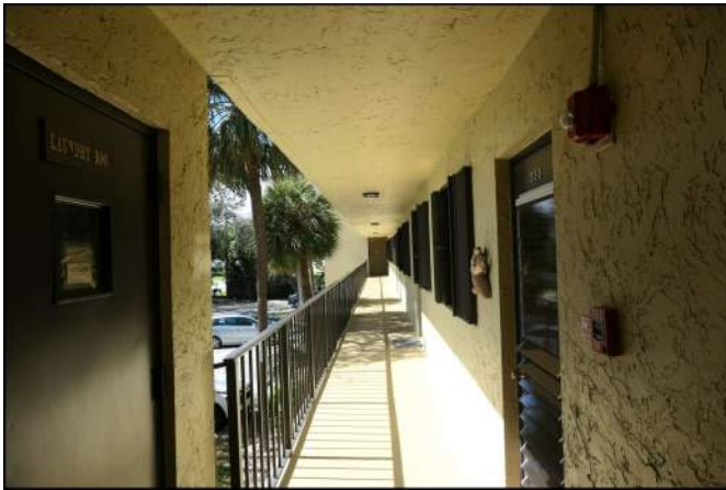
Photo 57 Building Structure and Envelope
