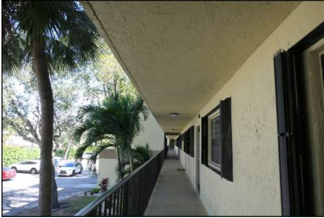
Photo 19 Building Structure and Envelope
