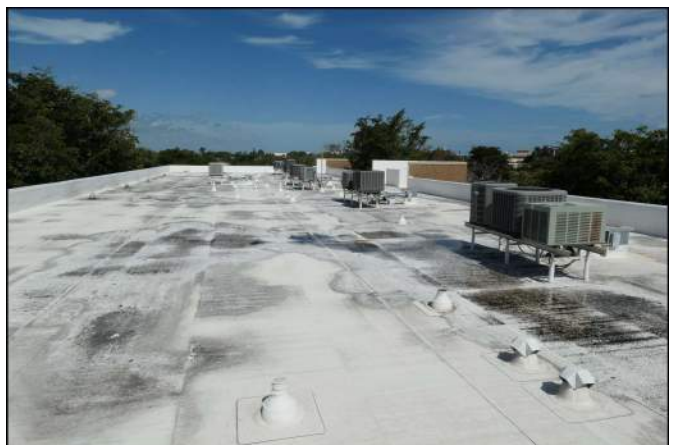
Photo 30 Building Structure and Envelope
