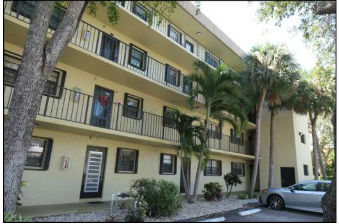
Photo 14 Building Structure and Envelope
