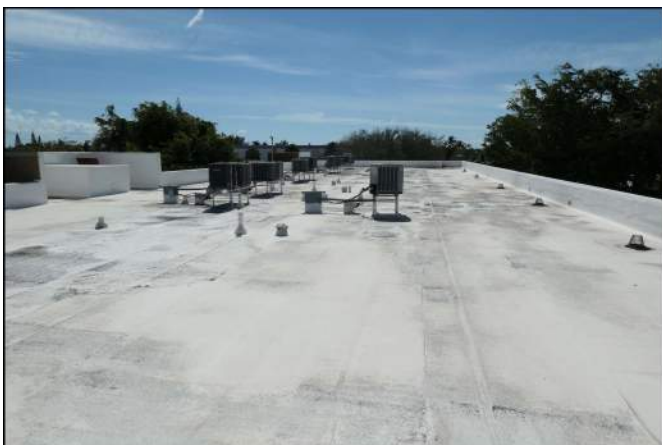
Photo 29 Building Structure and Envelope
