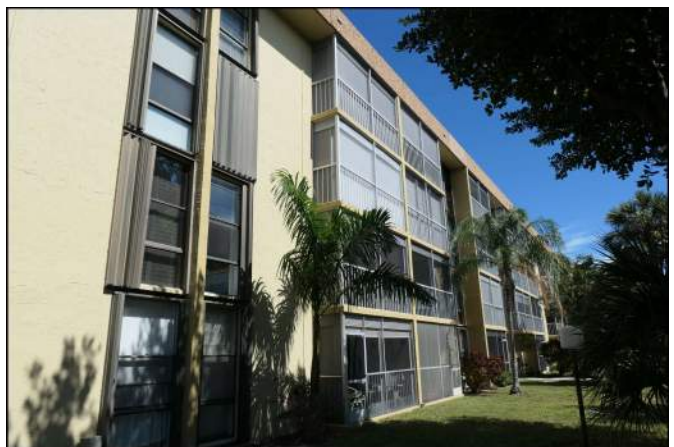
Photo 18 Building Structure and Envelope
