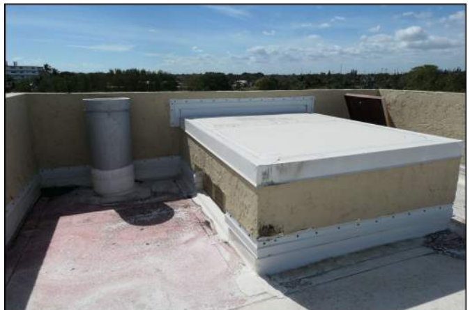
Photo 48 Building Structure and Envelope
