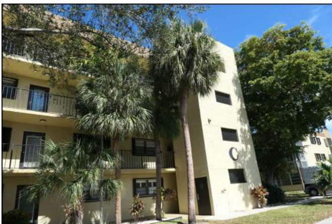
Photo 53 Building Structure and Envelope
