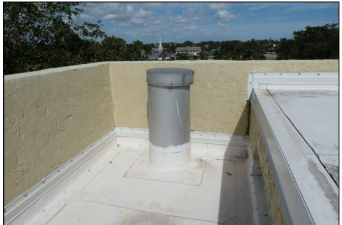
Photo 10 Building Structure and Envelope
