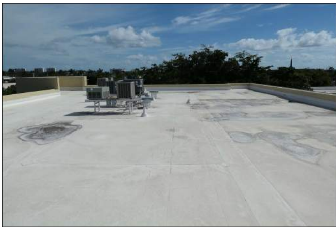
Photo 05 Building Structure and Envelope
