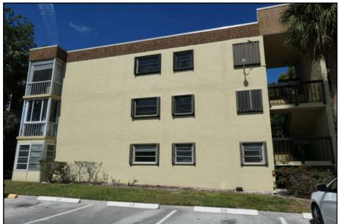
Photo 42 Building Structure and Envelope
