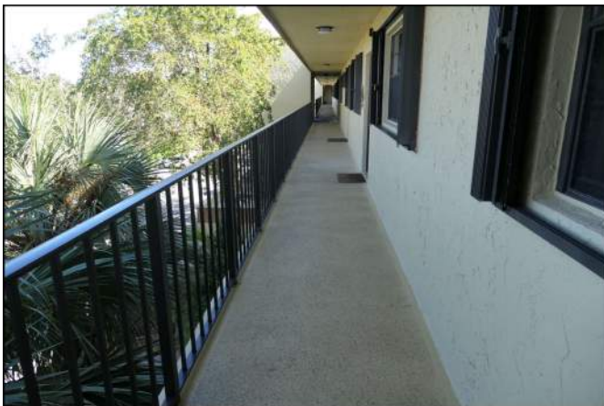
Photo 23 Building Structure and Envelope
