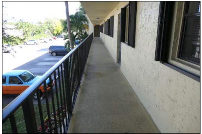
Photo 22 Building Structure and Envelope
