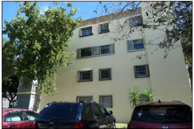
Photo 16 Building Structure and Envelope
