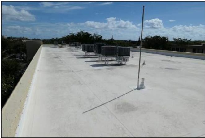
Photo 03 Building Structure and Envelope
