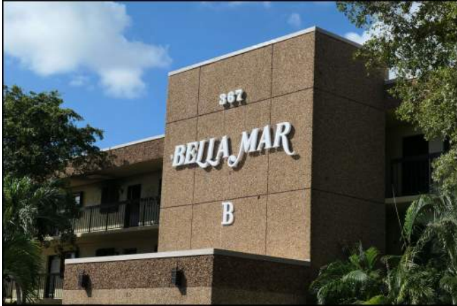
Photo 25 Building Structure and Envelope
