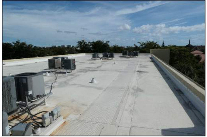
Photo 44 Building Structure and Envelope
