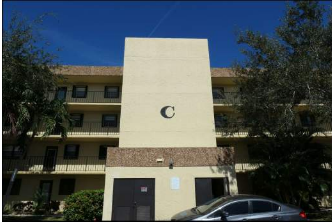
Photo 43 Building Structure and Envelope
