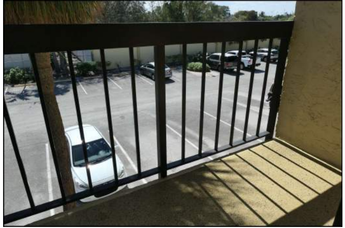
Photo 38 Building Structure and Envelope
