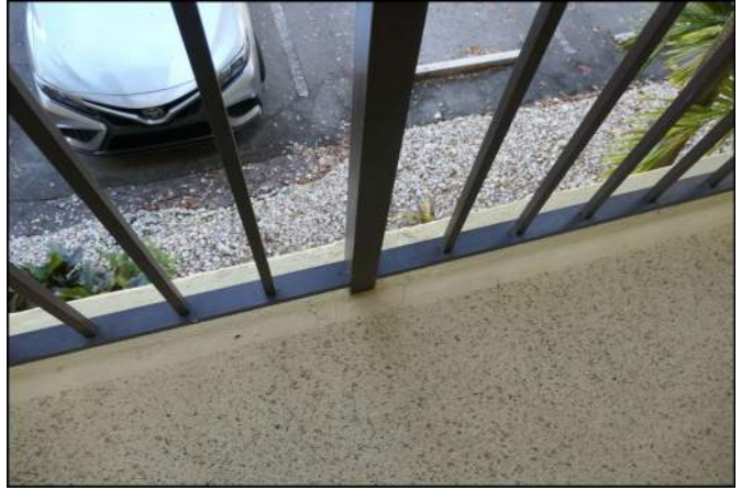
Photo 20 Building Structure and Envelope
