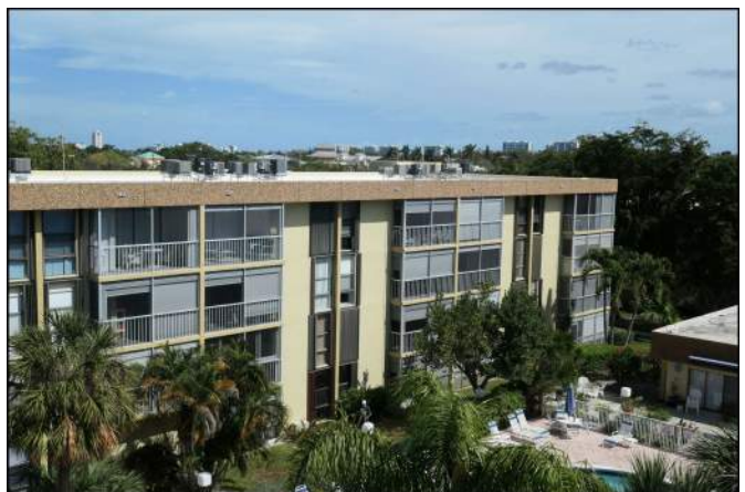
Photo 12 Building Structure and Envelope
