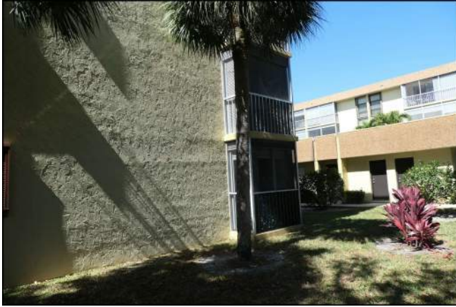
Photo 55 Building Structure and Envelope
