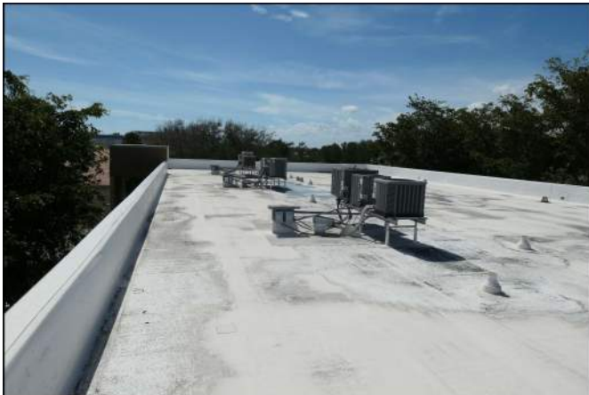
Photo 27 Building Structure and Envelope
